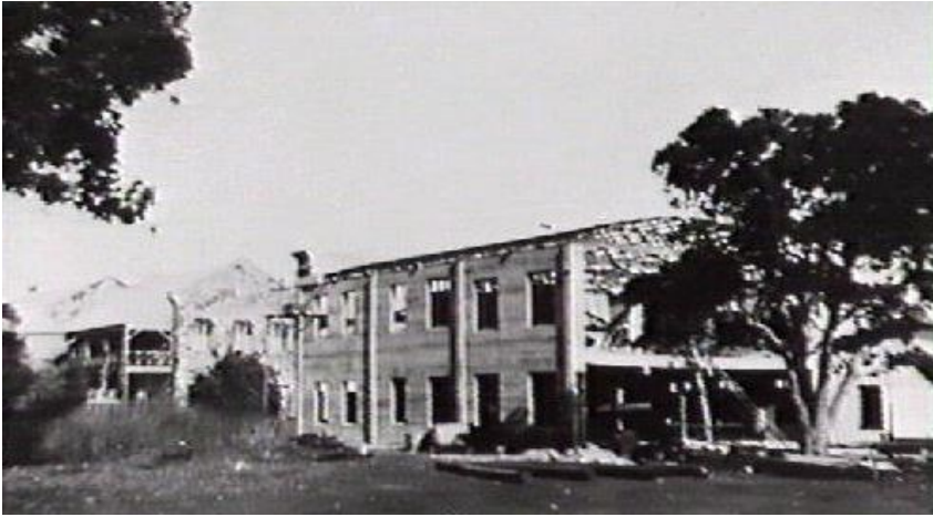
1929 – Star Theatre under construction. Image: FR Morris Collection, NT Library.
